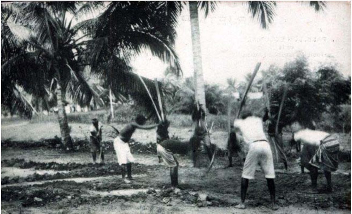
Photograph 18: Road construction was the most common form of prestación personal
